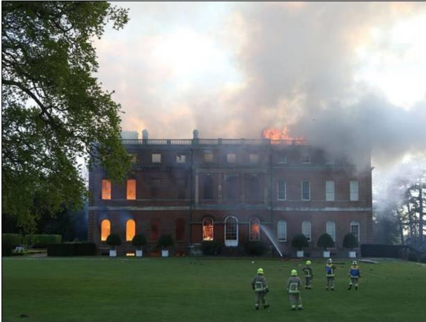
Clandon Park fire ( www.Independent.co.uk ). See AGM notice below
